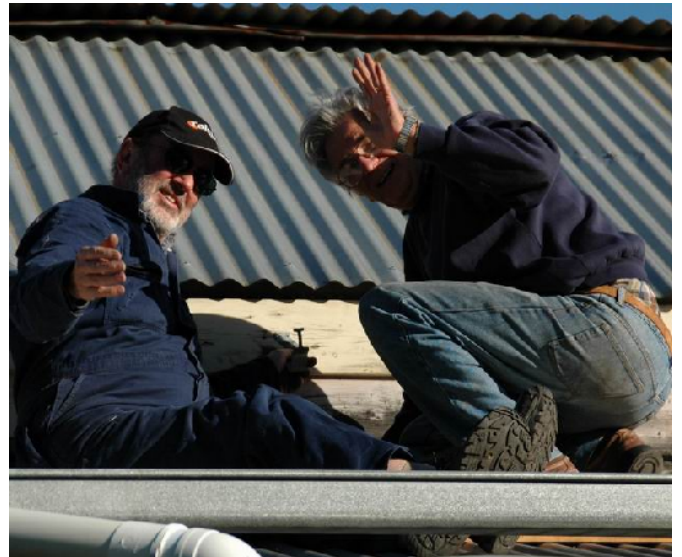
Daryl and Miles enjoying the sun (repairing the spouting).
